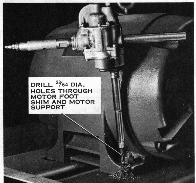
FIG. 12— DRILLING MOTOR FOOT, SHIM AND MOTOR SUPPORT
