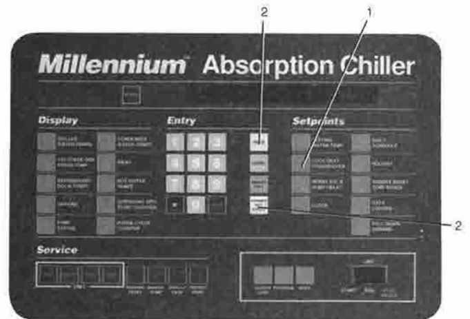
FIG. 6 - KEYPAD - PROGRAMMING "COOL/HEAT CHANGEOVER" SETPOINT
