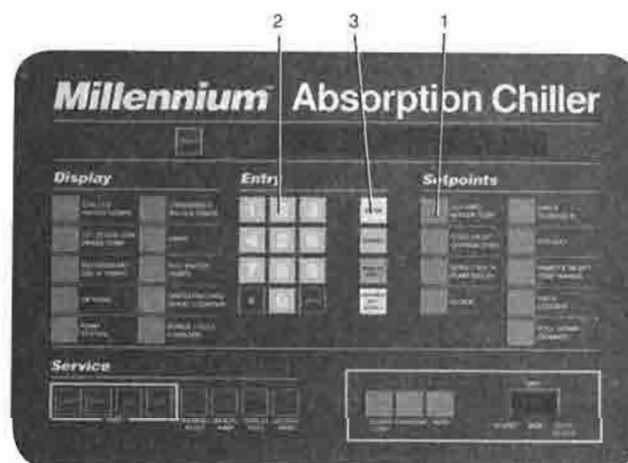
FIG. 5 - KEYPAD - PROGRAMMING "LEAVING HOT WATER TEMP" SETPOINT
