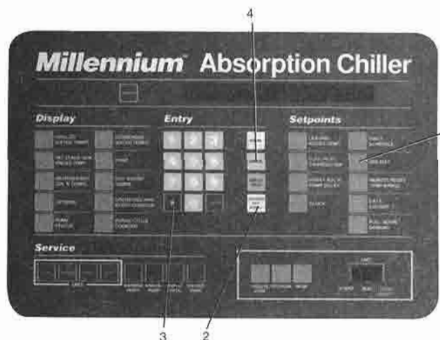
FIG. 9 - KEYPAD - PROGRAMMING "HOLIDAY" SETPOINT
